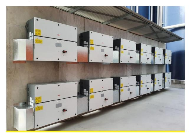
Huon Hoogesteger, Managing Director of Smart Commercial Solar, explains why FIMER inverter technology was his technology of choice for this project: "The FIMER PVS-100 fits perfectly for the MV (medium voltage) system size of this project. It is easy to install and fits within the inverter station that was specially designed and engineered by our team."
