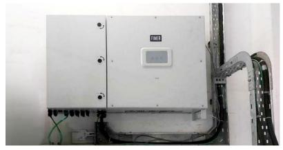
The PVS-50 system is designed for easy installation and reduced installation costs, with the power module and wiring box enclosed in a single compact chassis. It also has hinges and cam latches on the cover for easy interior access.
