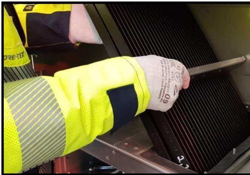
Image of a FIMER inverter repair
