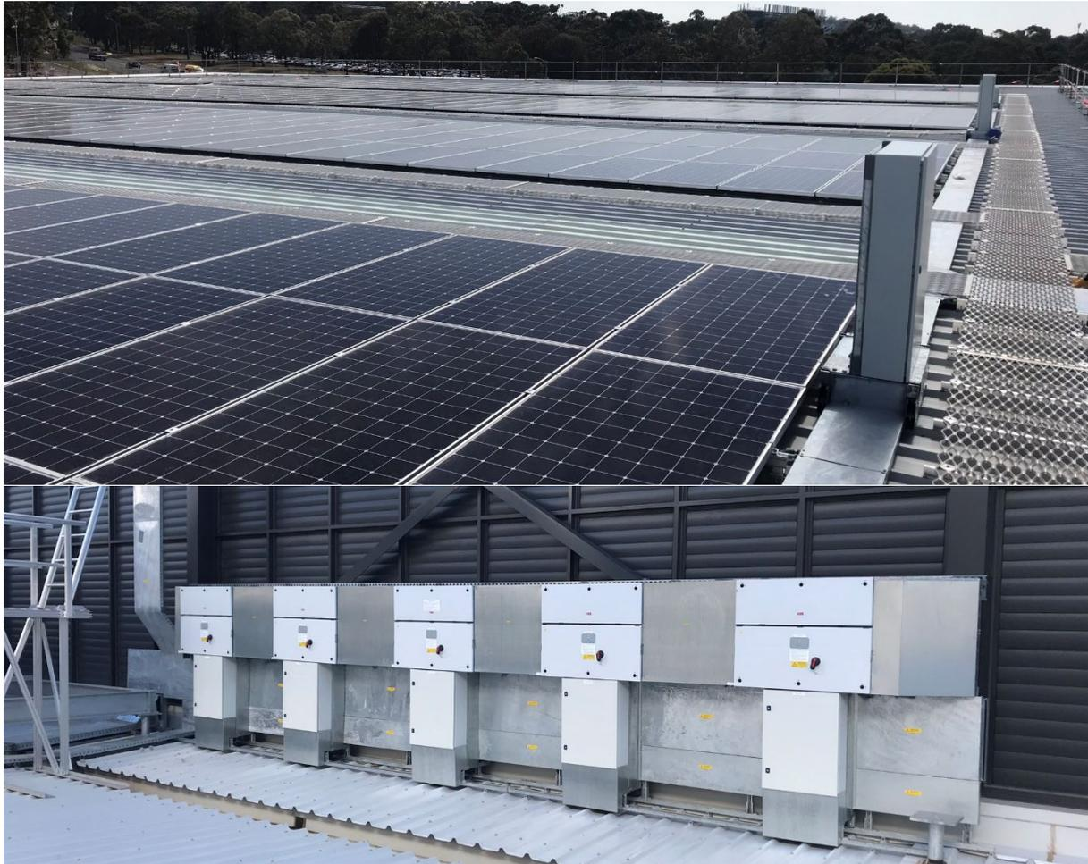
FIMER's five PVS-100-TL string inverters are located on the roof and built into a custom-made enclosure. The PVS-100 inverter, which is made in Italy, is ideal for this type of application where energy demand fluctuates, and the high power-rating of each inverter means that fewer units are required, reducing CAPEX, due to its high-power density and cuts OPEX as it is quick to install, easy to configure and maintain.
