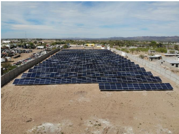
Saucillo city , 1 PV installations with PVS-120
