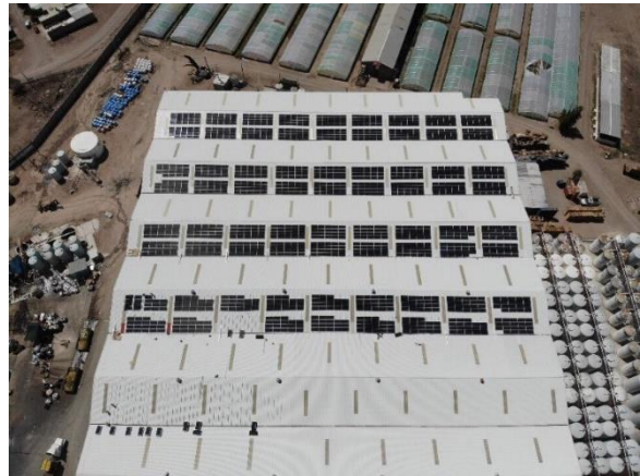
Naica , in Saucillo. Roof project with PVS-120
