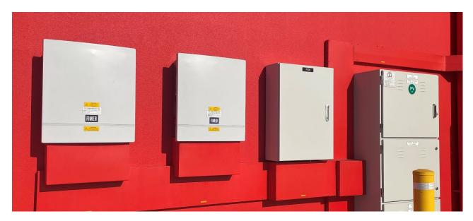
FIMER's PVS-10/33 is an Italian-made three-phase string inverter that comes in six power sizes, including 10kW, 12.5kW, 15kW, 20kW, 30kW and 33kW and is an ideal solution for large residential and commercial and industrial applications.
