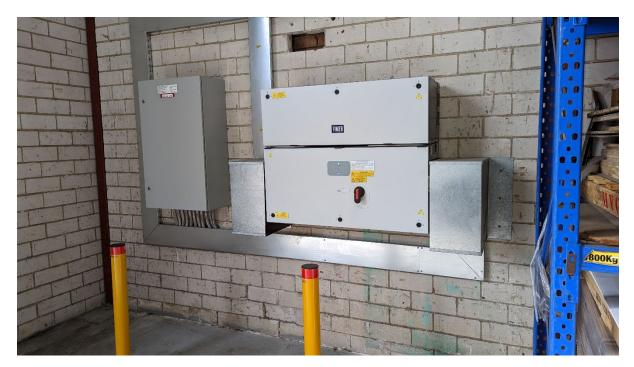
FIMER's PVS-100 is an all-in-one high-power string inverter. It is the best solution for businesses needing to maximise their investment return for large, decentralised roof-top installations. The PVS-100 inverter installed at Allprint Graphics has six MPPTs enabling greater design flexibility and energy yield, the system can also be ordered with two MPPTs for applications where the inverter is located a long way from the solar panel array.
