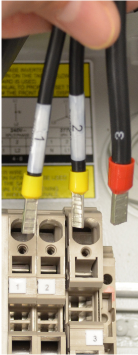
Figure 4 Remove AC wires from terminals 1, 2 and 3
