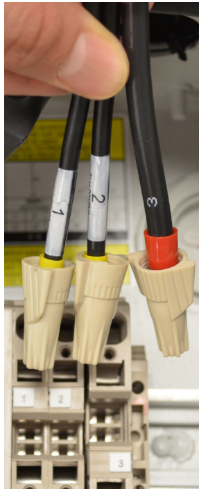
Figure 5 Secure the exposed wires using wire nuts
