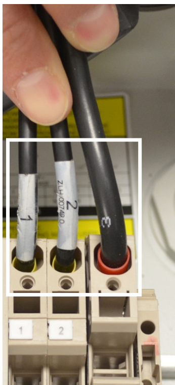
Figure 13 Wires labeled 1, 2 and 3 reconnected to terminals 1, 2 and 3
