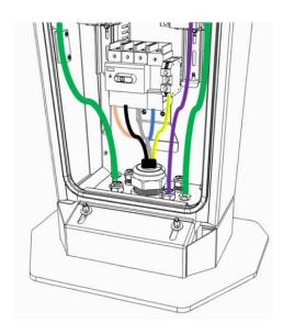
Once the top of the column is reached, the end of the Ethernet cord should be plugged into the appropriate Ethernet port:
